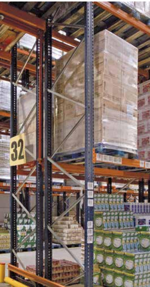
Selective pallet racking system with pallets handled from their 800 mm side
