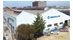
Plant in Buenos Aires, Argentina
