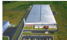
Plant in São Paulo, Brazil
